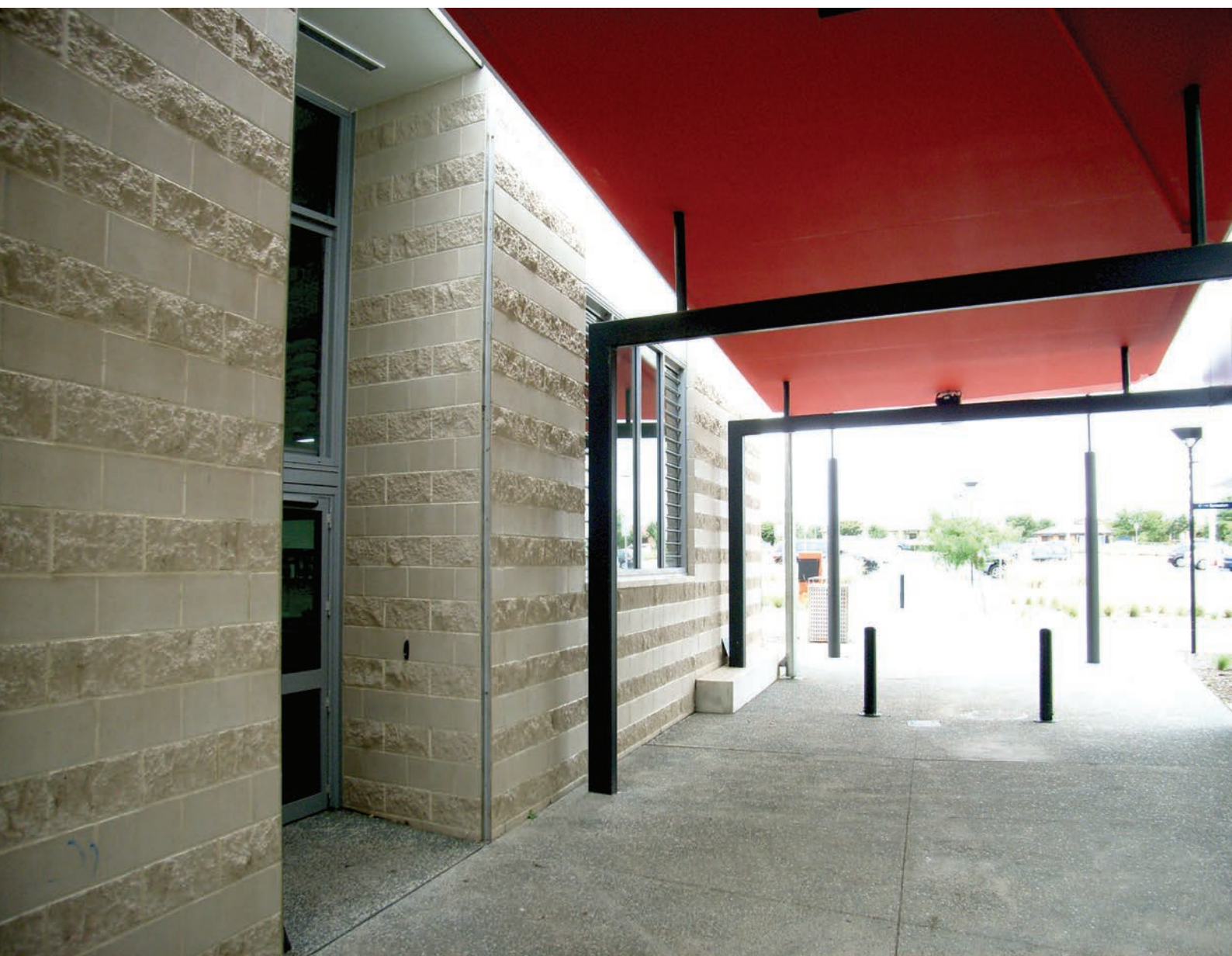
Split and smoothface block wall in Opal White
